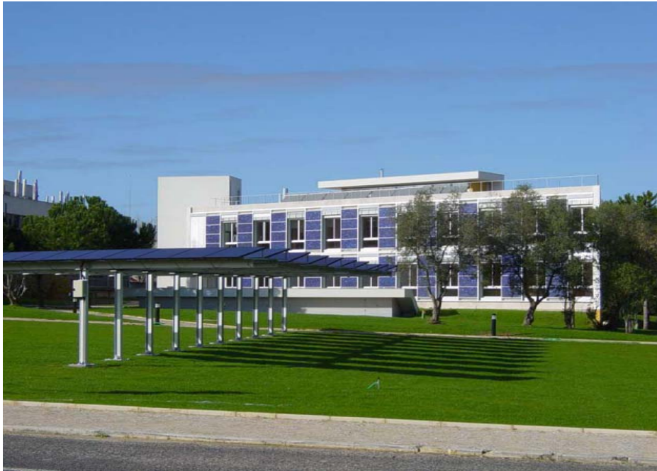
SolarXXI building, showing a 100 m 2 PV facade
