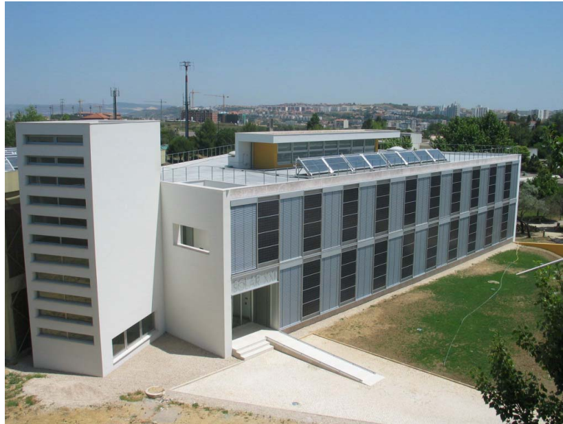
View of the SolarXXI building
