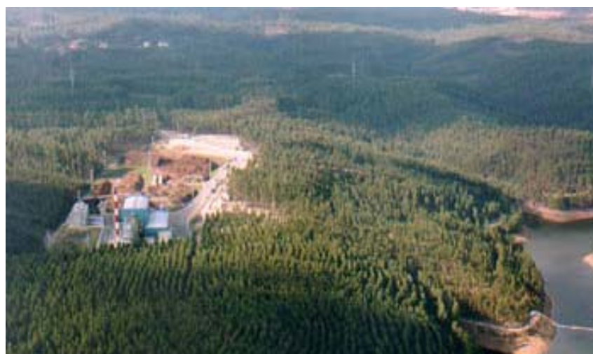
Fig. 1 - Mortágua Power Plant ( BIOMASS - Forest Residues Plant - Energie-Cités )
